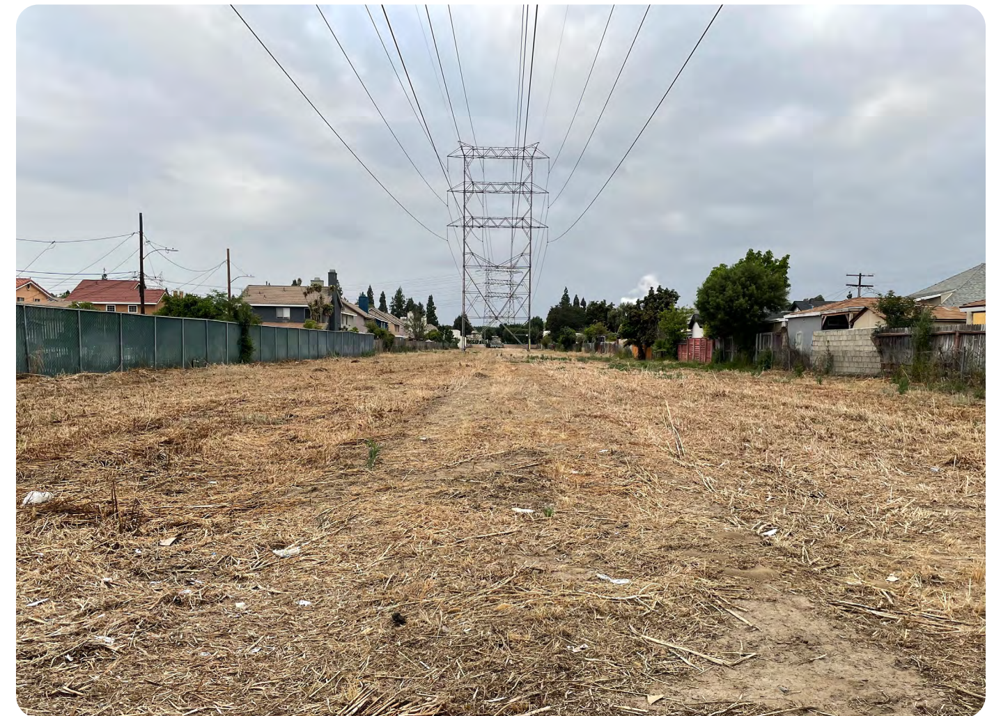
Image: Utility Corridor near Jefferson Street and Hayter Avenue
