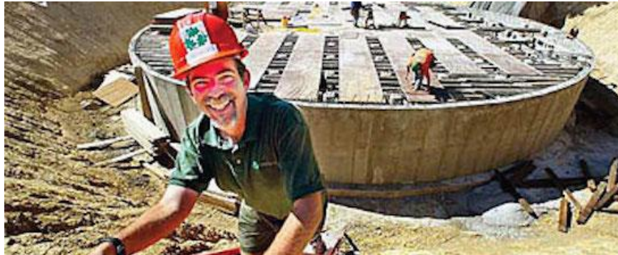
Photo Credit: LA Times, Andy Lipkis inspecting TreePeople's cistern which can capture 216,000 gallons of stormwater
