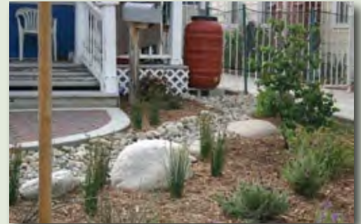
A home on Elmer Avenue in Sun Valley features a rain barrel, permeable paving and native landscaping.
