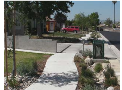
These before and after photos show some of the Northeast San Fernando Valley's neighborhood retrofit on Elmer Avenue. Improvements include curbs and gutters, parkway bioswales and native trees.
